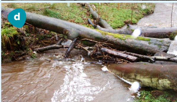
Figure 2: Example locations for leaky barrier installation. (a) Floodplain – promote temporary storage on adjacent land (Photo: Mark Wilkinson, JHI). (b) In-ditch – slow flow and trap sediment in agricultural ditches (Photo: Addy et al. 2025). (c) Ephemeral stream – barriers in small, seasonally flowing streams to intercept runoff (Photo: Martyn Roberts, JHI). (d) Woodland – barriers using natural woody debris (Photo: Nicholson et al. 2012).
