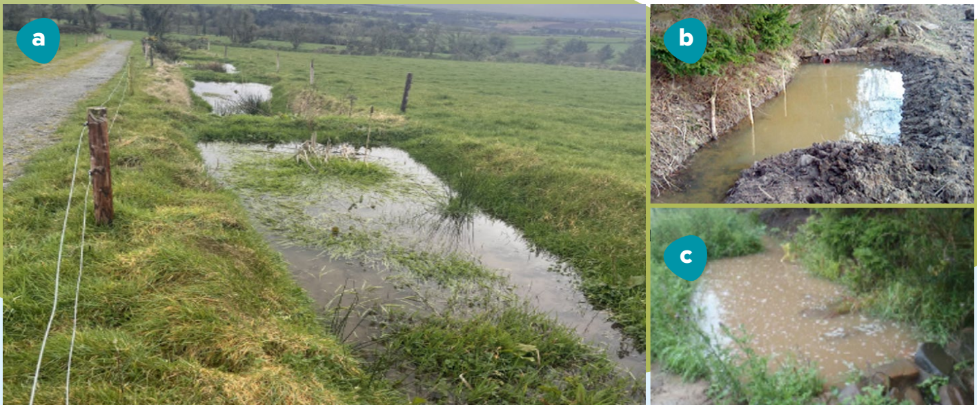
Figure 2: Examples of in-ditch sediment traps. (a) Series of traps installed in a field ditch (photo: Farming for Water EIP). (b–c) In-ditch sediment traps located upstream of a runoff storage pond; (b) photo: Mark Wilkinson (JHI), (c) photo: Newcastle University.
